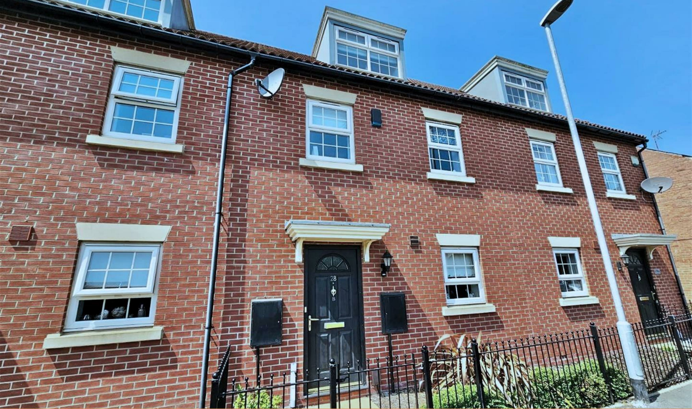
The Twitchell, Sutton-In-Ashfield, NG17 5DA
